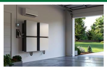
The base capacity for residential systems ranges from 10 to 13.5 kWh, which can power an average home. Your energy needs will vary depending on the appliances you have, how often they run, and how much backup power you want. Appliances such as air conditioners and water heaters may drain the capacity quicker, and you may want to disconnect them during an outage. Make sure to check with Dunn Energy about specific system requirements.
